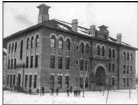
In May 1901, while acting president of BYA, GHB urged construction of a building for the Church Normal Training School, with a gymnasium on the upper floor.
